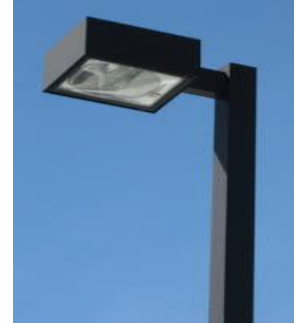
Example: Downward lighting
